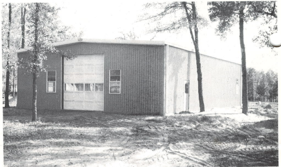
Spacious new garage constructed.
